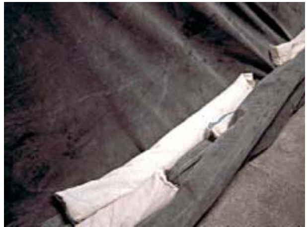
7.4 Sand snakes to ensure air tight fumigation
