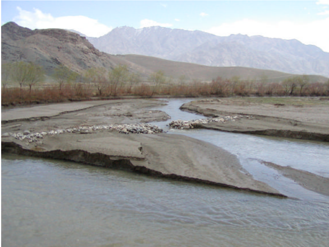
Figure 4.1: Typical loose masonry water diversion structure
