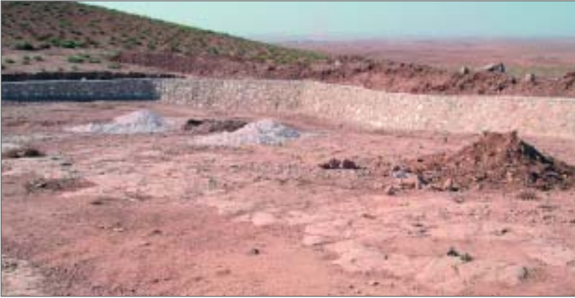
Small water reservoirs were built at project sites in Lebanon, to collect and store runoff water for use by livestock.
