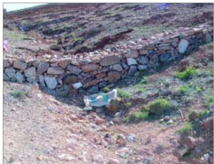
Low-cost check structures have proved effective in stopping runoff water and retaining the soil it carries.
