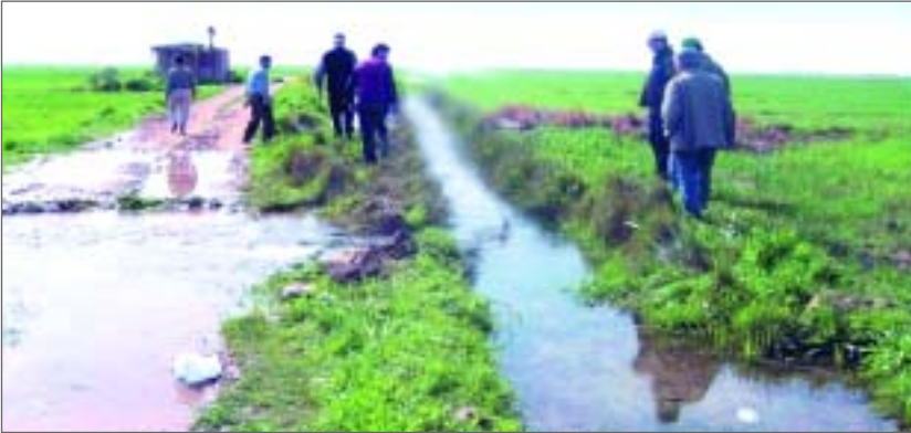
Poorly managed water conveyance structures and practices in the basin area: the bank of this irrigation ditch has been cut, to convey water across the road to another field – creating problems of excess runoff.
