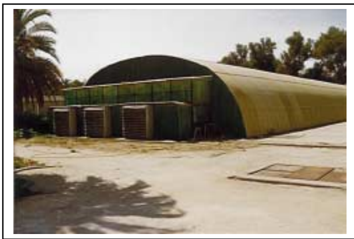
Positive-pressure evaporative cooling system at the Research Station of PAAAFR, Kuwait
